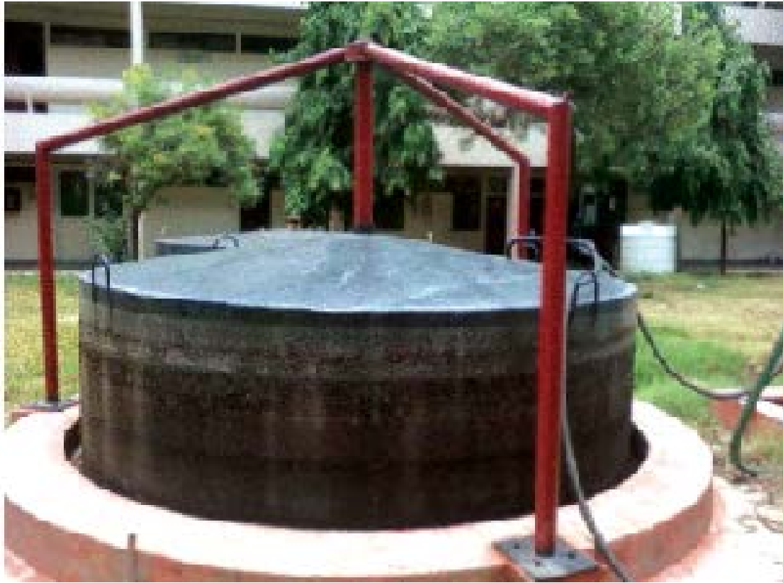
Gobar Gas Plant uses cattle dung to produce energy
